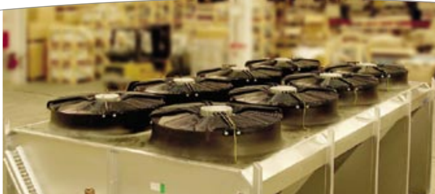
Meticulous control of fans saves energy and keeps noise and draft at a minimum.
